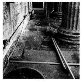
Fig. 15 Town Hall, record photograph showing the podium's asphalt covering, together with an area where the primary Belper stone has been exposed to view. Photograph, Gareth Lewis, 2003; courtesy, Birmingham City Council
